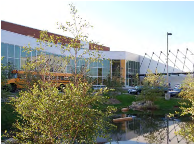
A welcoming entry creates a sense of safety and community in this urban setting
