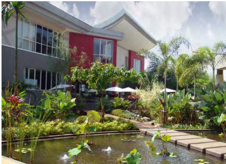
Above: Gardens and a pond serve as learning opportunities for Sinarmas students - note the large over-hangs that shade the windows and doors from the intense local sunlight
